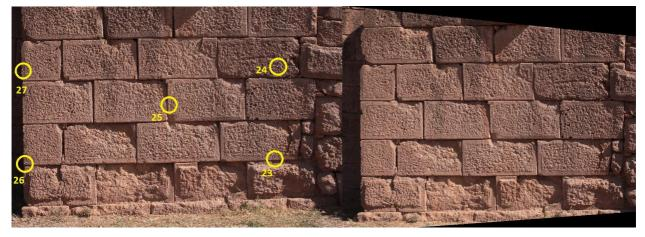
Figure 5a. The original image to be rectified with the five targets on the wall (left). The rectified image (right.
